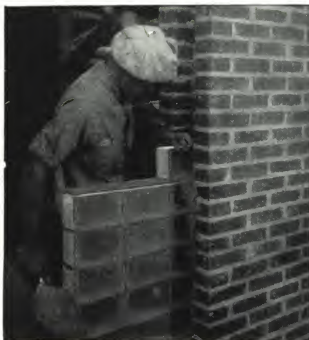
Insulux Glass Blocks are light in weight and are of a size that is convenient for the mason to handle. They lay up quickly in the same manner as other masonry units.
